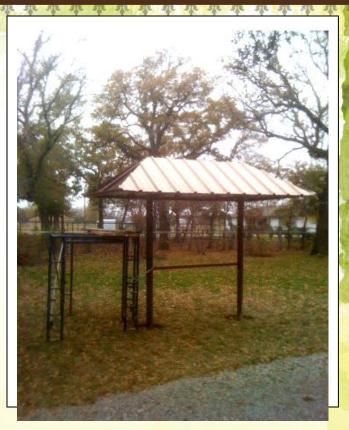
Under Construction — Map Display Case Kiosk: Work has begun on the plot map display case kiosk with steel awning and frame. The base will be 6x12' and stone work will surround the support posts. The display case already has been constructed and will be mounted when the kiosk stone masonry and base have been completed.
